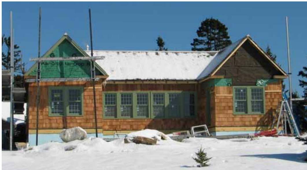
Above top: House on cribbing. We moved it, built a foundation under where it had been, and moved it back. Project architect Richard Manzo and I felt it important that it stay exactly where it was. Now, Windswept is much stronger. We reinforced most of the truly daring framing (2 x 4 rafters on 30" centers). It has been on an insanely exposed site for almost 100 years and was pretty straight. Maybe we don't need that code! Above bottom: House in snow with green windows. The color change on the outside comes from the book, which talked about dark green trim, but also talked about colors to match the sea outside. We opted for a muted green, and our new shingles will soon be gray. Photos courtesy of Knight Associates.
